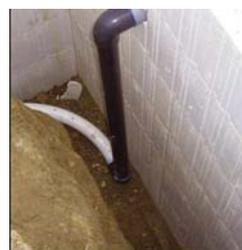
**LE TUYAU RIGIDE VERTICAL DOIT ÊTRE POSÉ OU BLOQUÉ SUR LE BÉTON DU RADIÉ SINON LE POIDS DU REMBLAI DÉTÉRIORERAIT L'ENSEMBLE ET OCCASIONNERAIT DES FUITES.**
